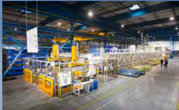
Hot forming plant in Gliwice
